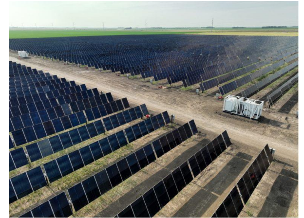
Double Black Diamond Solar Project Under Construction 800 MW
